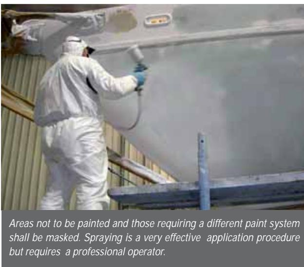
*Areas not to be painted and those requiring a different paint system shall be masked. Spraying is a very effective application procedure but requires a professional operator.*
