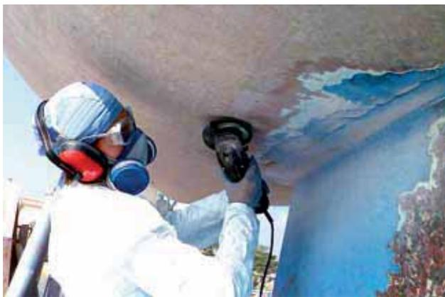
**3** Smoothing with an elliptical planing machine (outfitted with heat-resistant blades) and subsequently disc sanding with rotary or orbital disc sanders.
