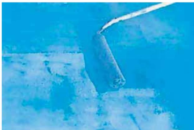
Before proceeding with the application of the primer, check the surface and, if necessary, sand with fine grade abrasive paper.
